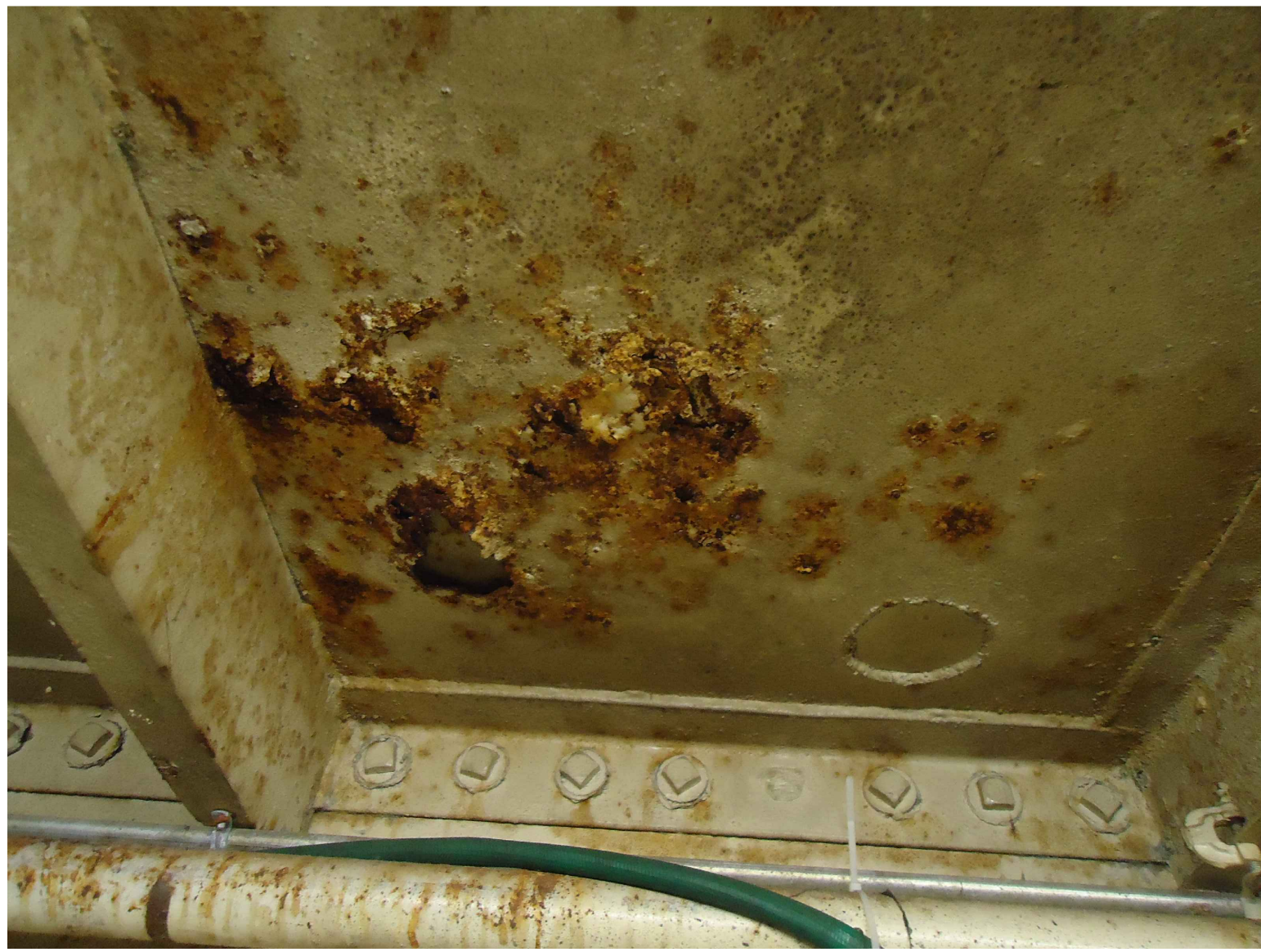
2 DECK PLATE DAMAGE NEAR A14
