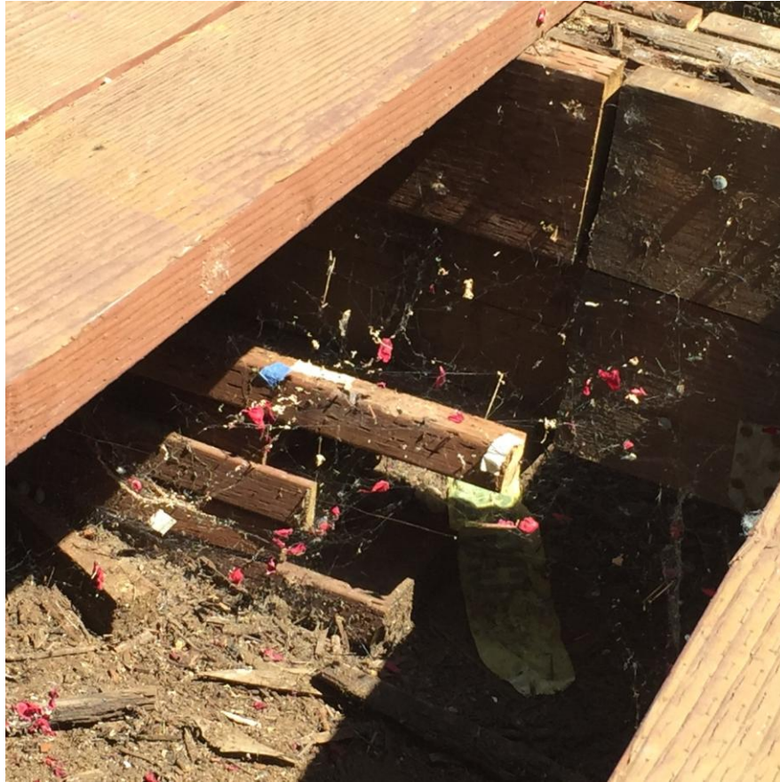
C line exposed spliced joists with blocking underneath.
