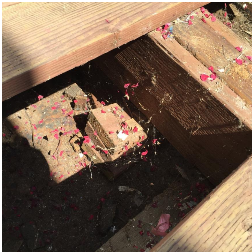
Close up of joists showing blocking intended to support joist
