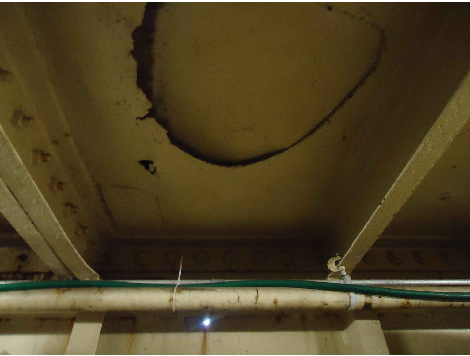
3 DECK PLATE DAMAGE NEAR D15
