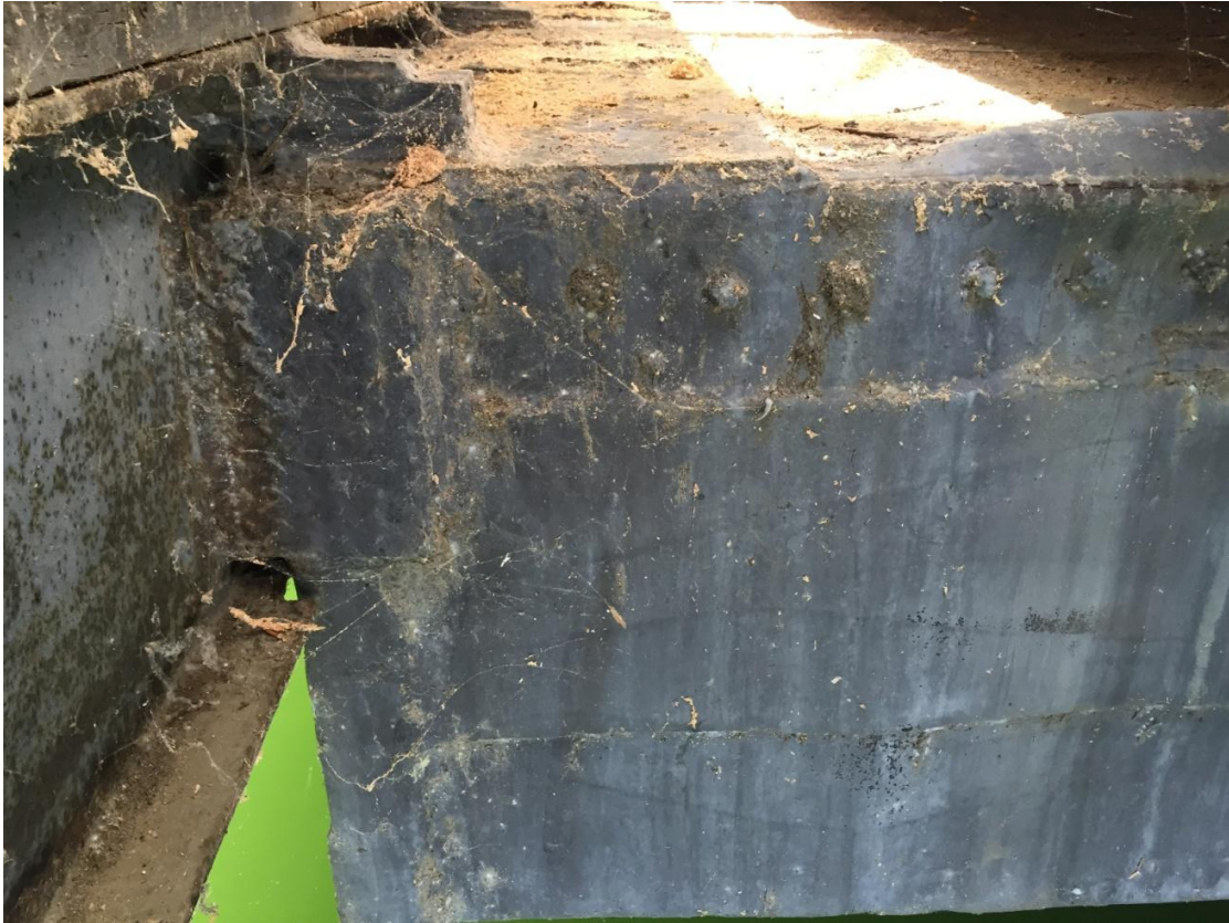
Underside of decking along E line showing I beam connection to ballast tank
