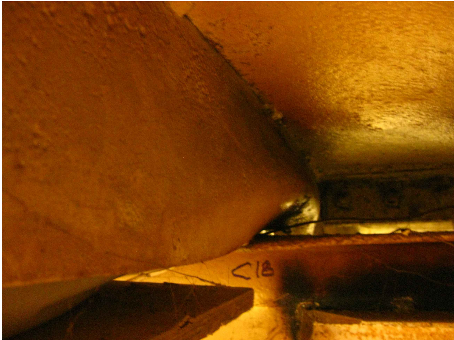
9 CONNECTION DAMAGE AT C18
