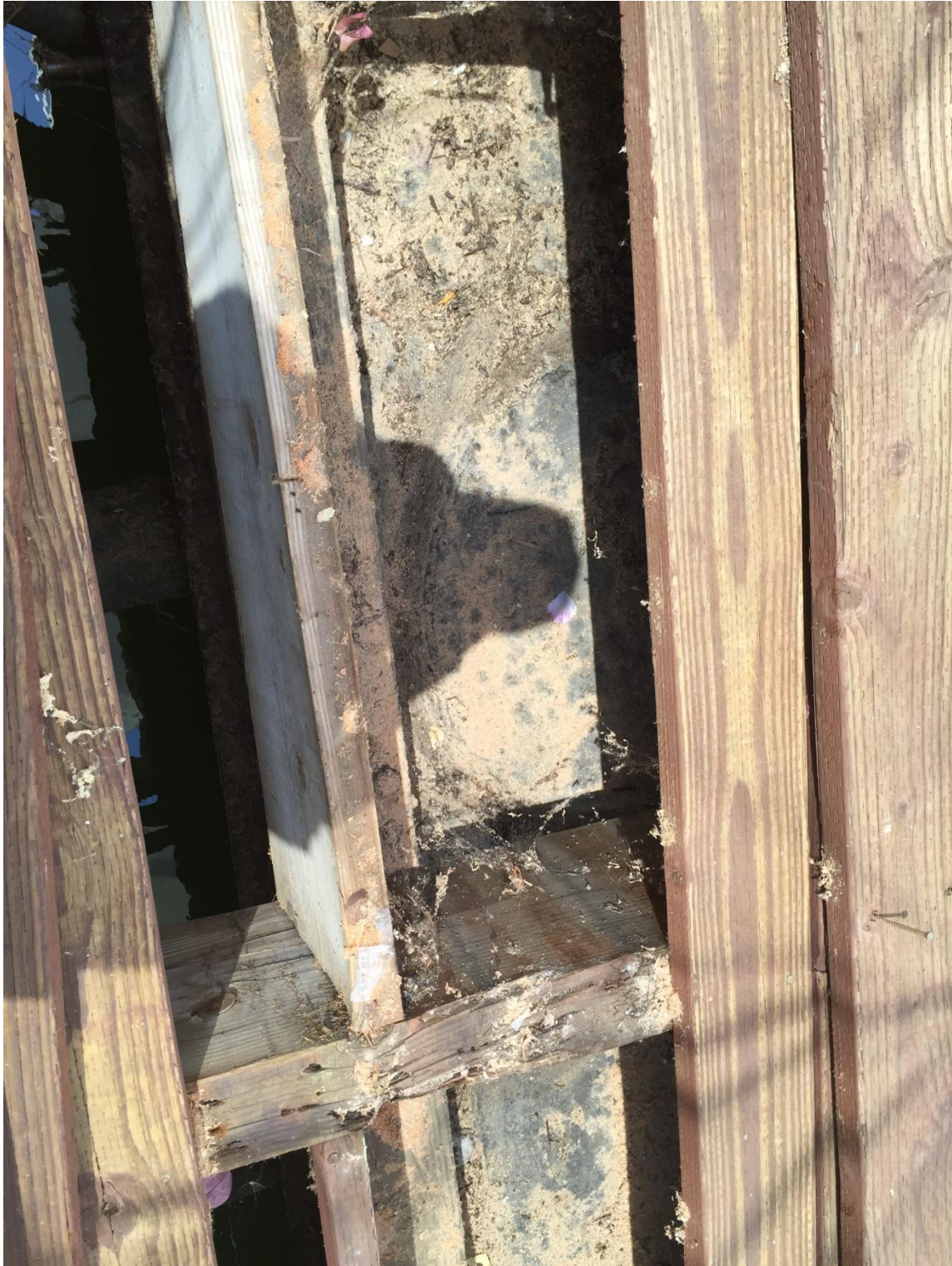
Close up of E 38 line area showing condition of joists.
