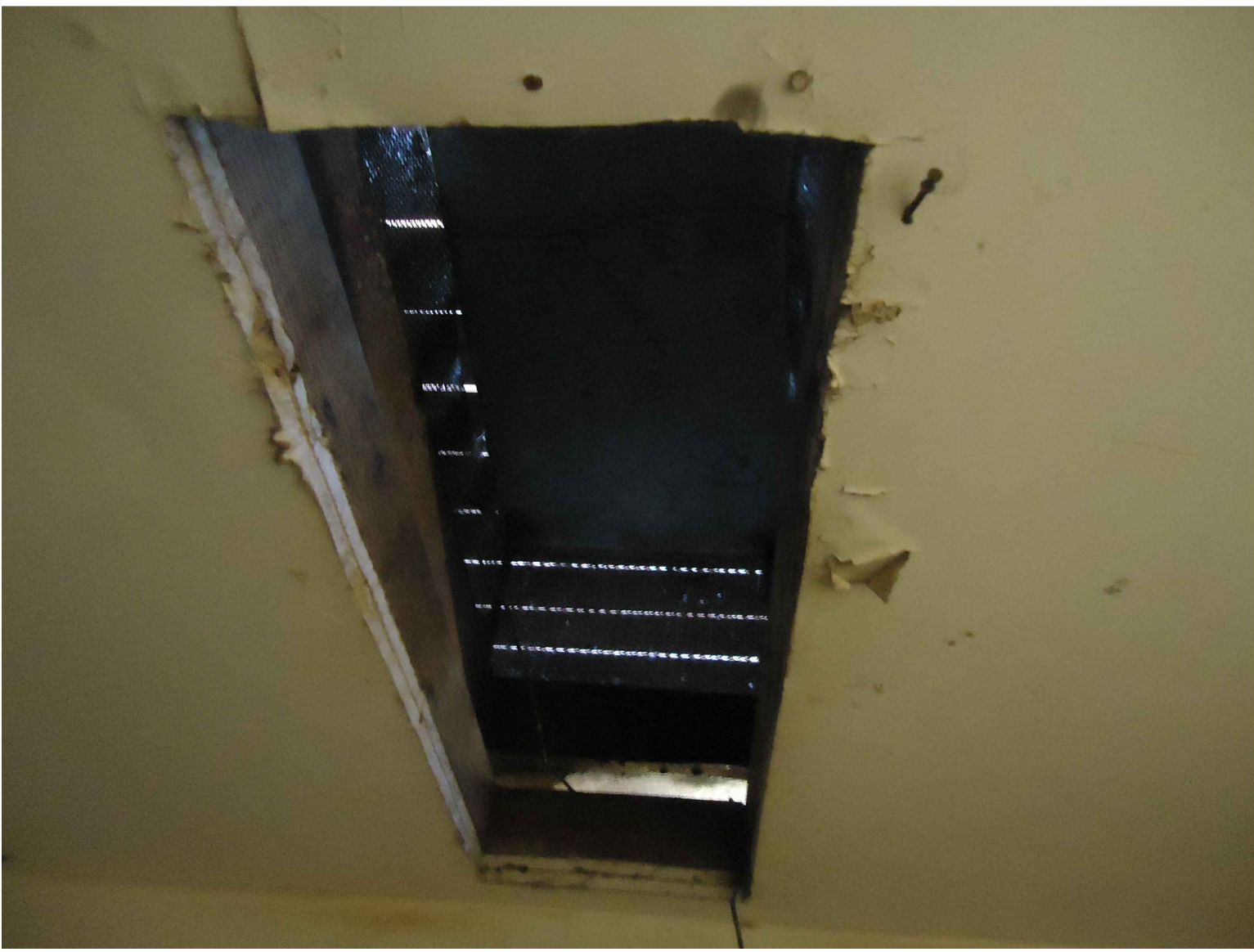
4 BOILER MAKE-UP AIR OPENING NEAR D36
