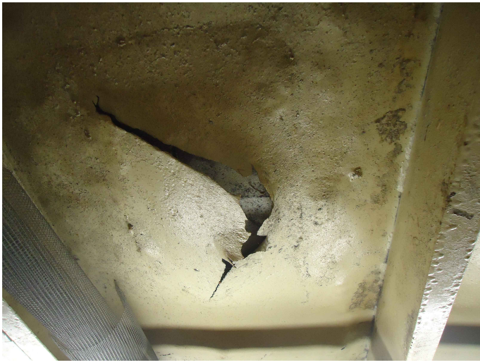
1 DECK PLATE DAMAGE NEAR D15
