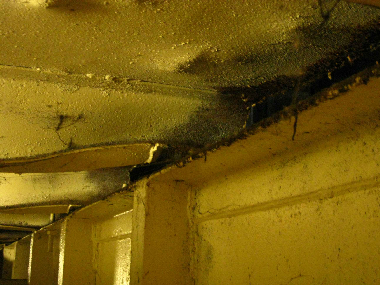
7 CONNECTION DAMAGE AT C8 THROUGH C10
