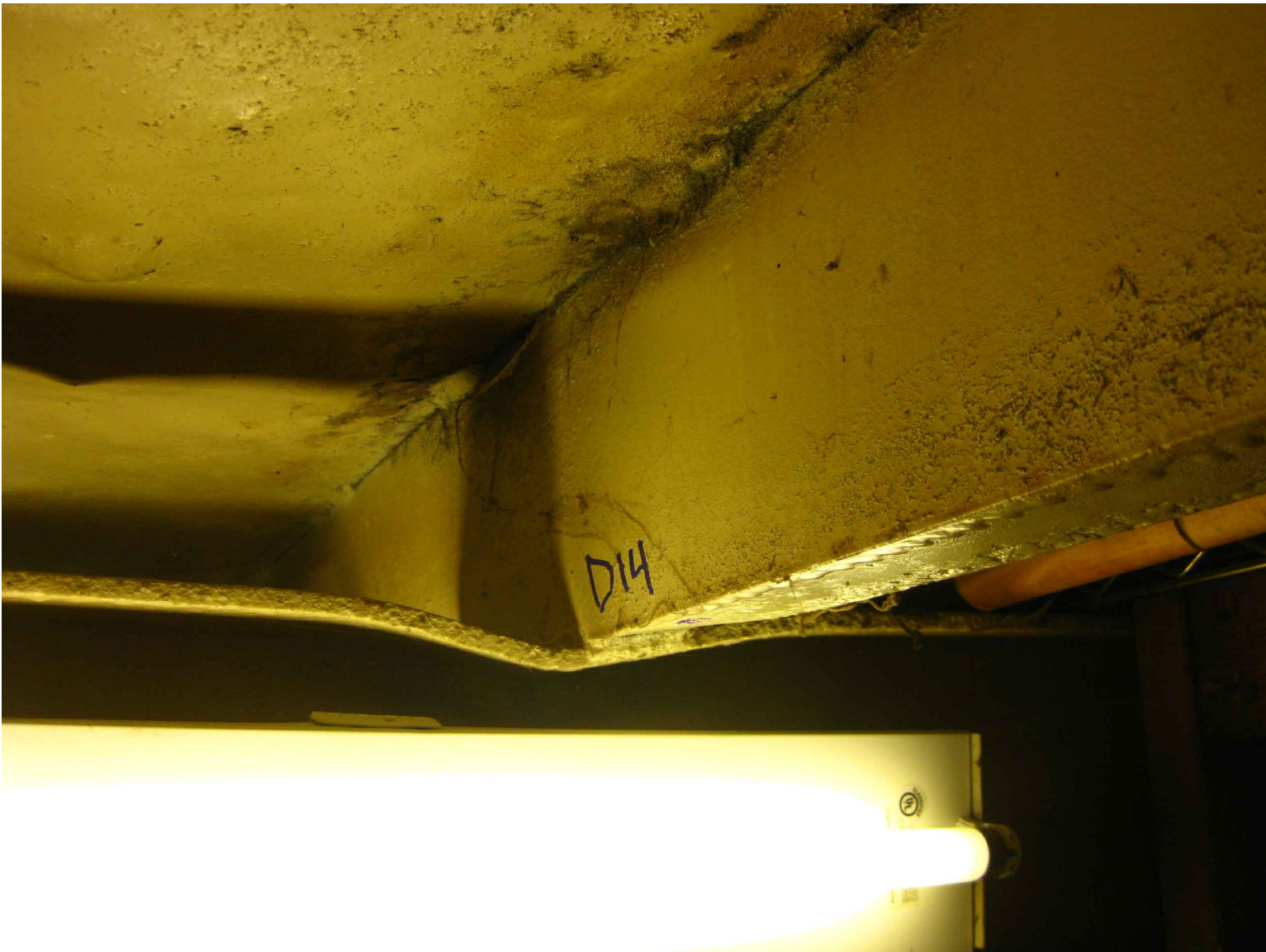
12 CONNECTION DAMAGE AT D14
