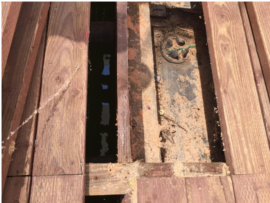
Close up of E 37 line opening showing threaded plug
