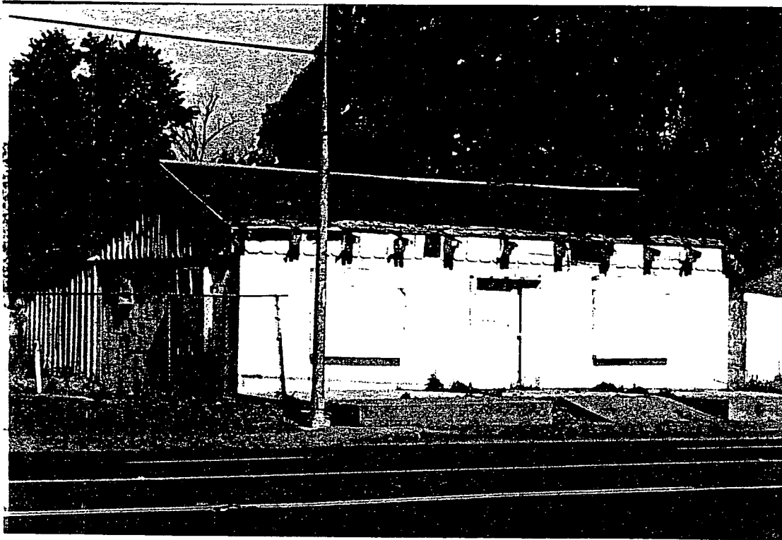
A deteriorated and sagging roof, damaged exterior building materials, and other exterior damage characterize this boarded-up structure on Marysville Boulevard.
