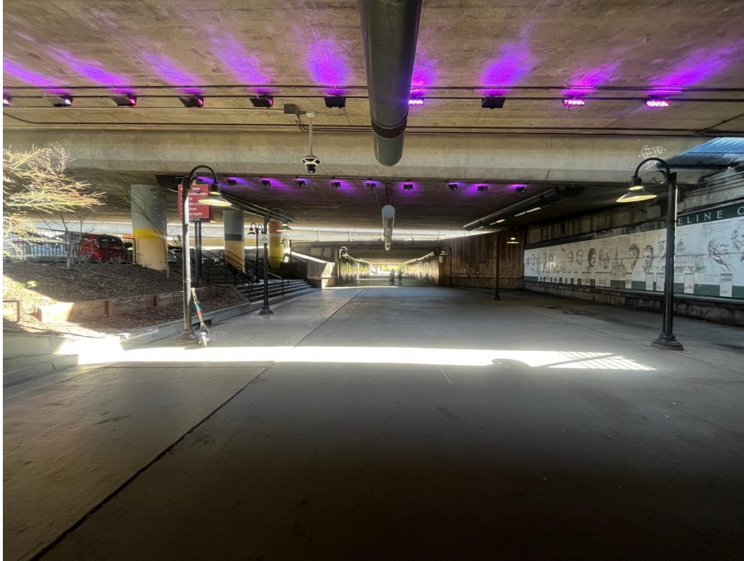
Figure 14: West side of the pedestrian tunnel, facing east, February 2026.
