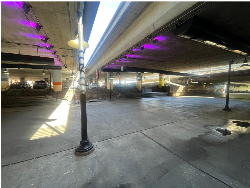
Figure 17: Pedestrian tunnel and adjacent parking lot, facing north, February 2026.
