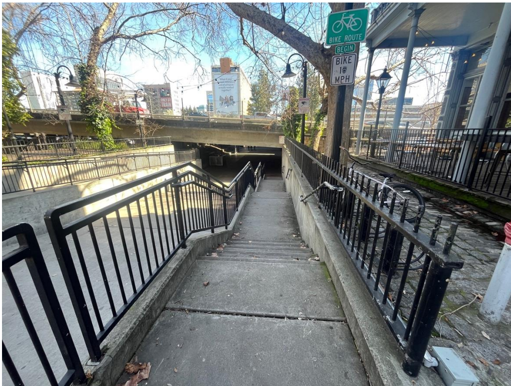
Figure 11: Stairs at the Old Sacramento entrance to the pedestrian tunnel, facing east, February 2026.
