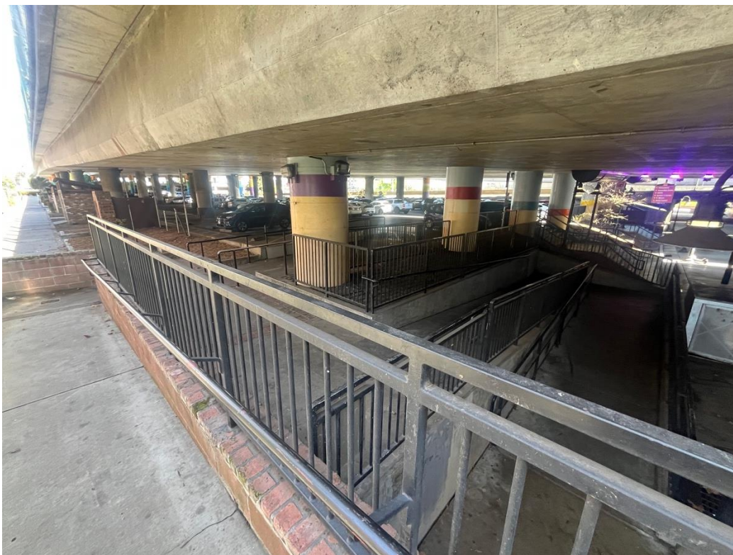
Figure 13: ADA ramp and adjacent parking lot, facing northwest, February 2026.
