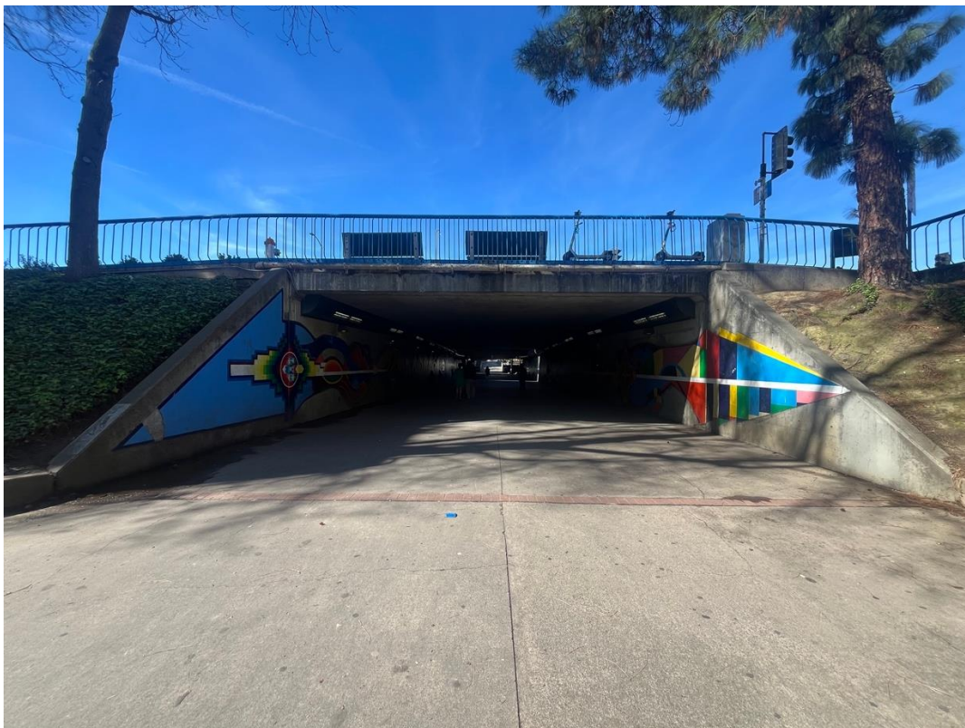
Figure 28: East entrance to pedestrian tunnel, facing west, February 2026.
