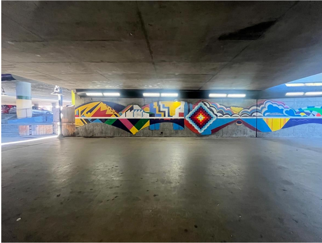
Figure 31: Portion of the northern wall of the Royal Chicano Air Force mural, facing north, February 2026.
