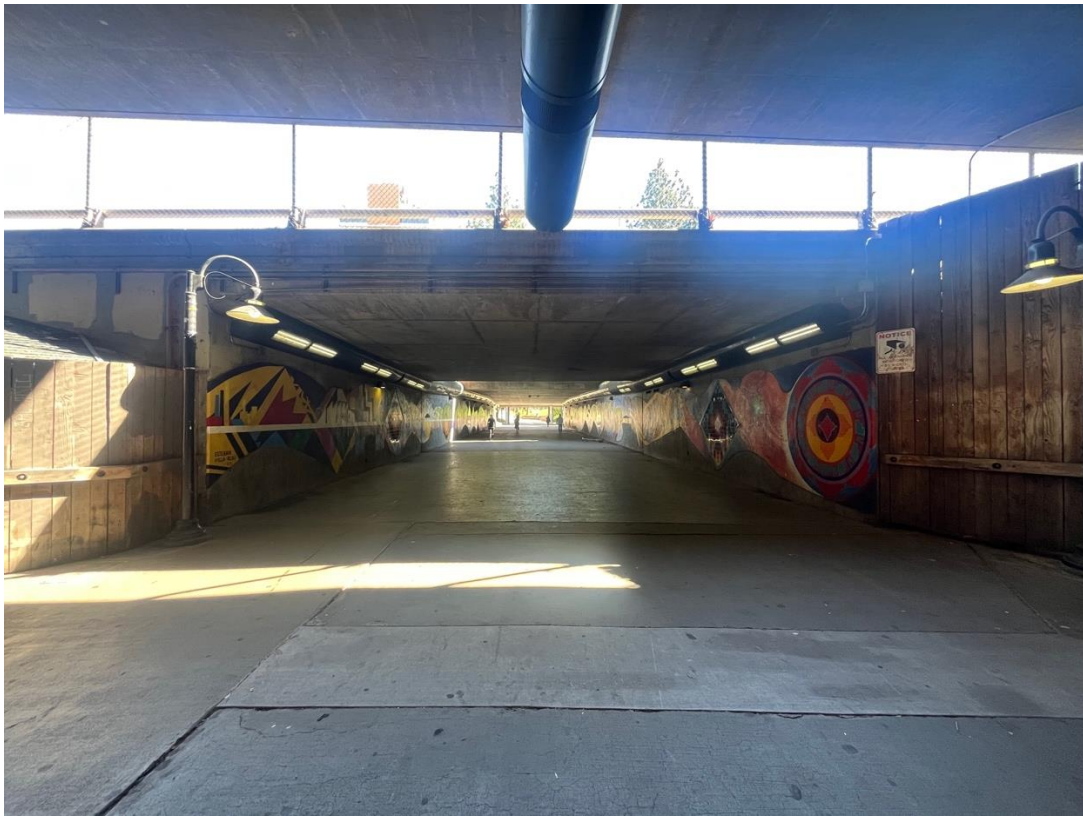
Figure 23: East side of the pedestrian tunnel, facing east, February 2026.
