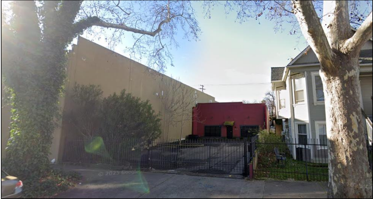
Figure 2: Existing Conditions – D Street
