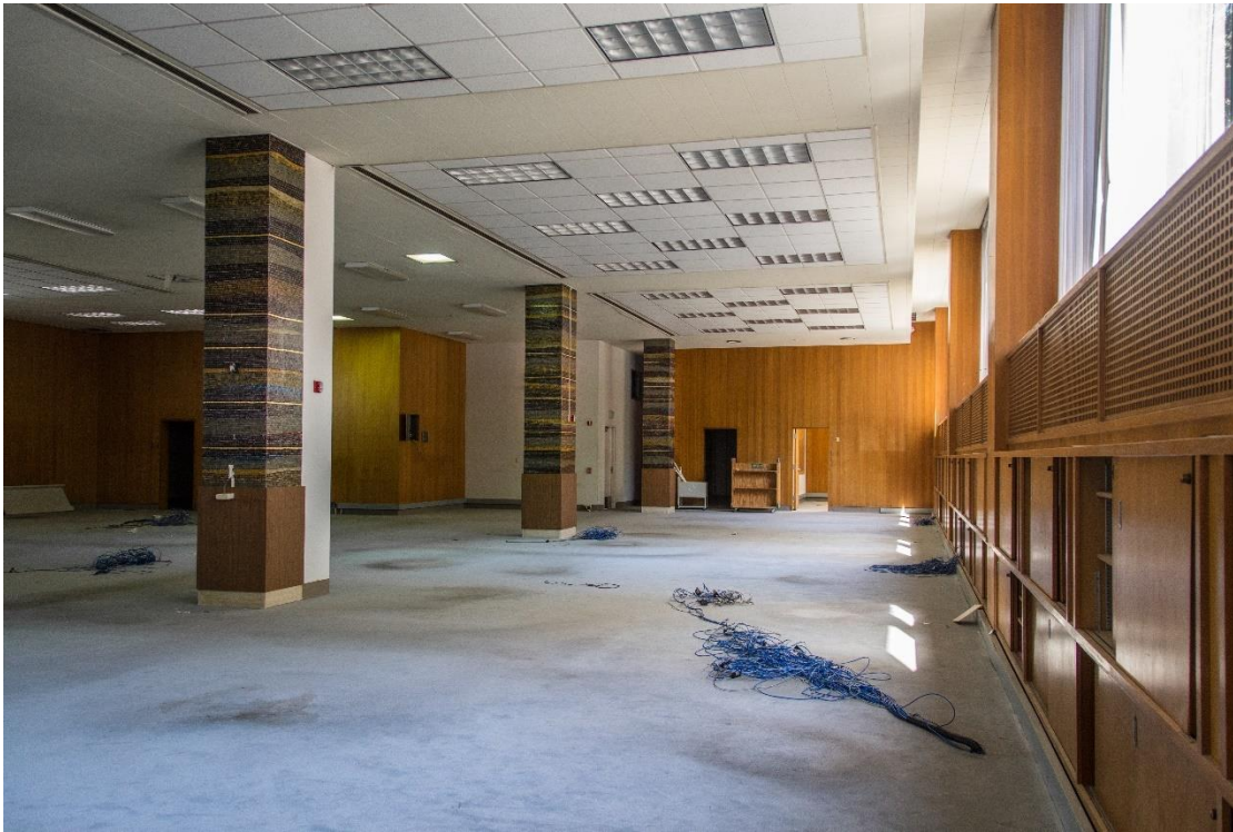
Mosaic tile columns with teak wood bases. The cabinetry on the right is teak as well.
