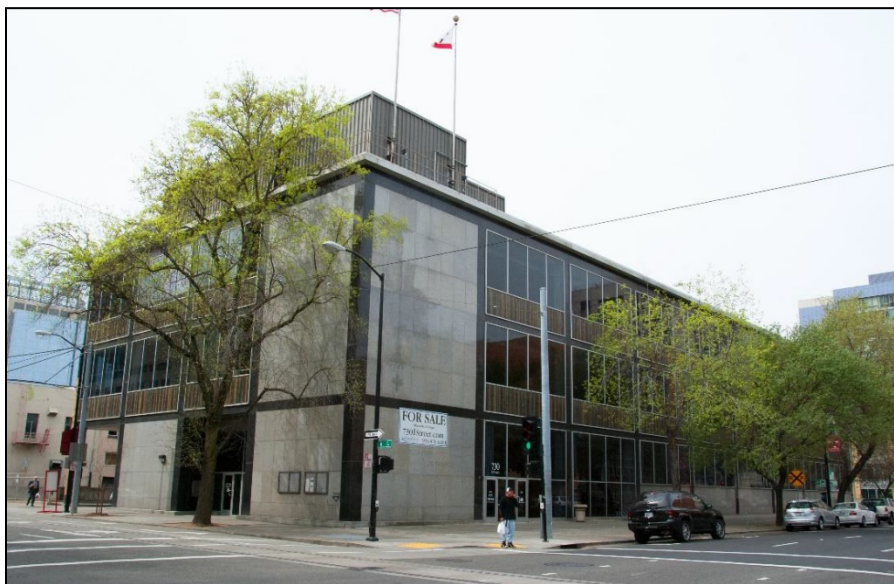
Figure 1: Bank of America Building at 730 I Street
