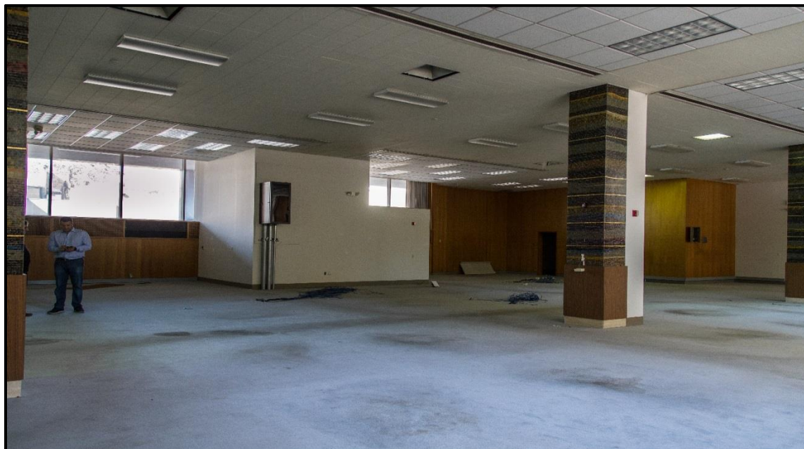
Ground floor office space, view to the southwest.
