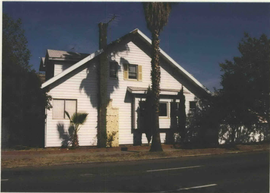
1631 26 th STREET SOUTH ELEVATION
