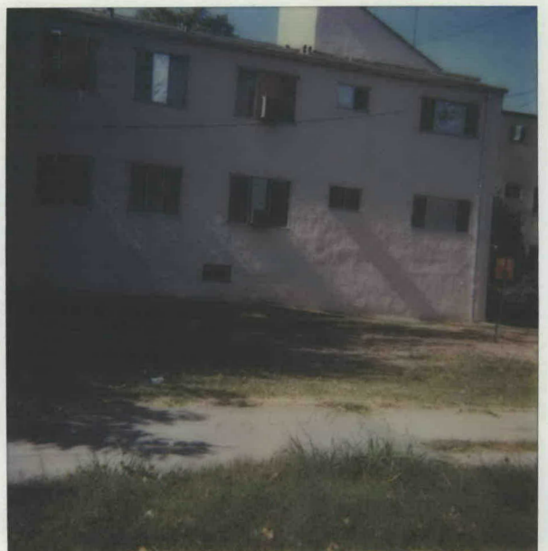
Vacant Rear Lot North of 1631 '0' St. New Construction Site
