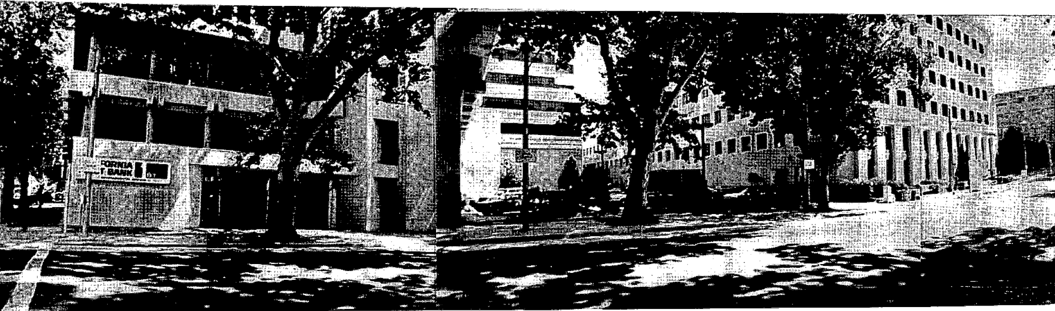
VIEW LOOKING EAST FROM GARAGE - ALONG 7th STREET
