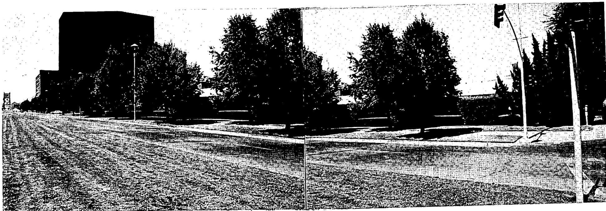
CAPITOL MALL VIEW OF GARAGE-LOOKING NORTHWEST
