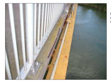
PHOTOGRAPH 1 – Spalling of the deck panel edge beyond the handrail. Note the exposed reinforcing bar.
