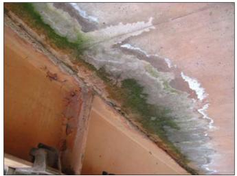
PHOTOGRAPH 2 – Typical staining on the bottom of a deck panel at the location of a joint seal.
