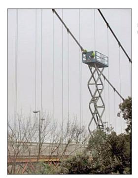
PHOTOGRAPH 1. Access to upper portions of most vertical suspender ropes using a manlift.
