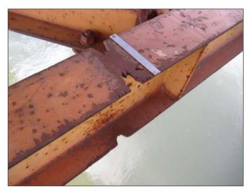
PHOTOGRAPH 3 – Damage to the stiffening truss lower strut at L53'.
