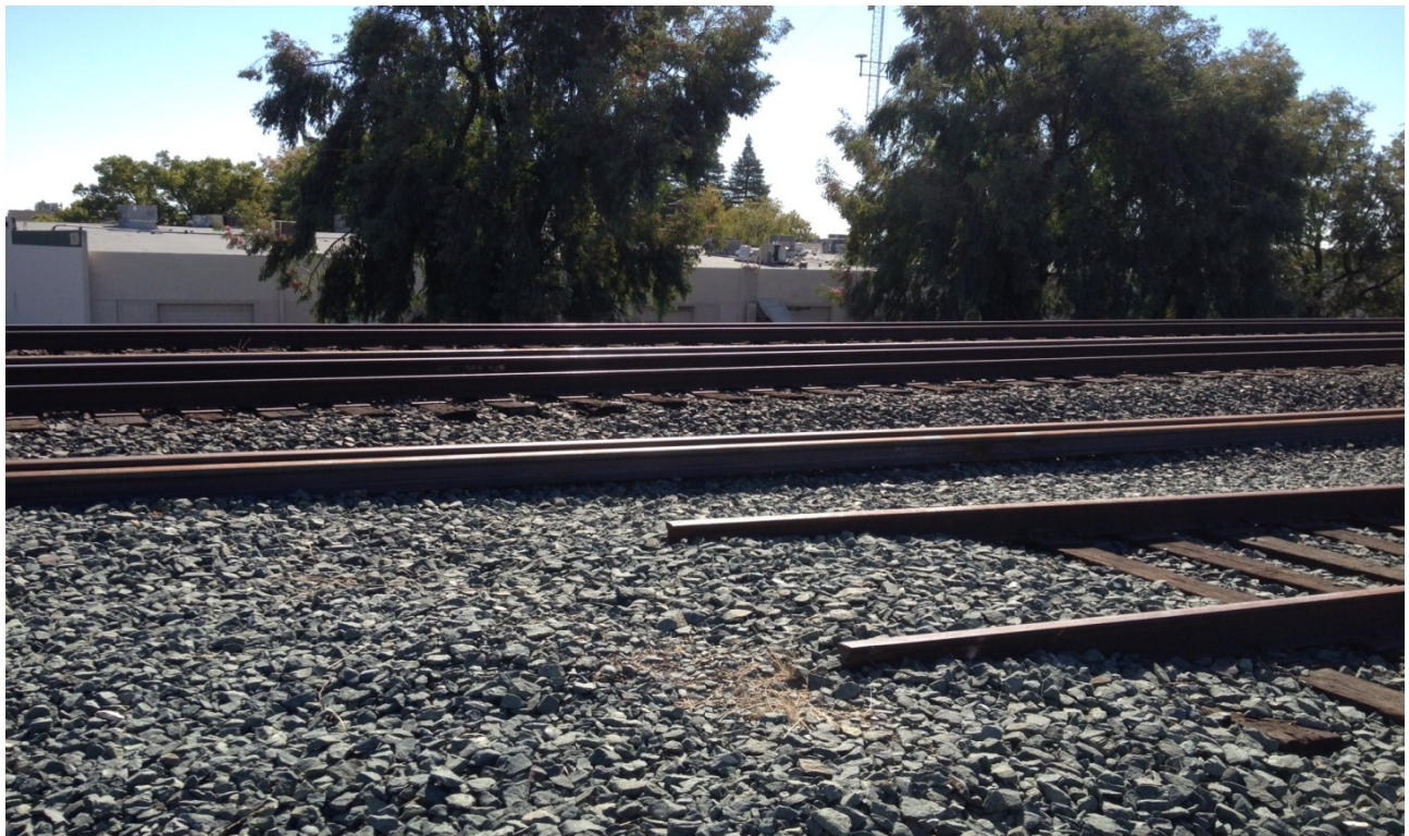
Photo 1C – Disconnected Rail Spur
