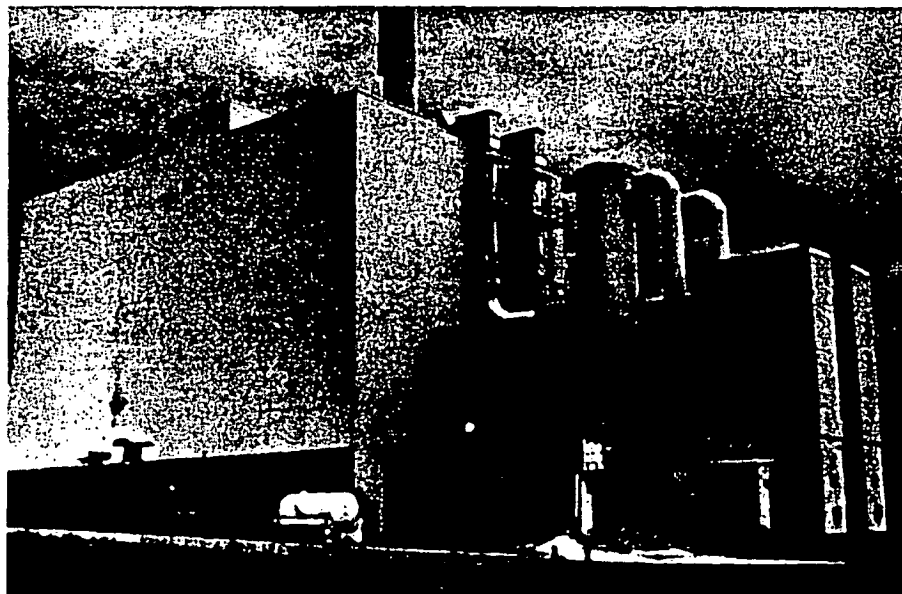
The waste-to-energy facility in Jackson County (Michigan) suffered a problem common to many MSW incinerators in the past few years—uncertainty over ash disposal. Operation at the 200-TPD mass burn plant began in October 1987, but was stalled for about eight months when the state initially classified incinerator ash as a hazardous waste. The state ultimately ruled ash to be a special waste, thus allowing the facility to resume disposing of its residue in a special cell at the county landfill.
