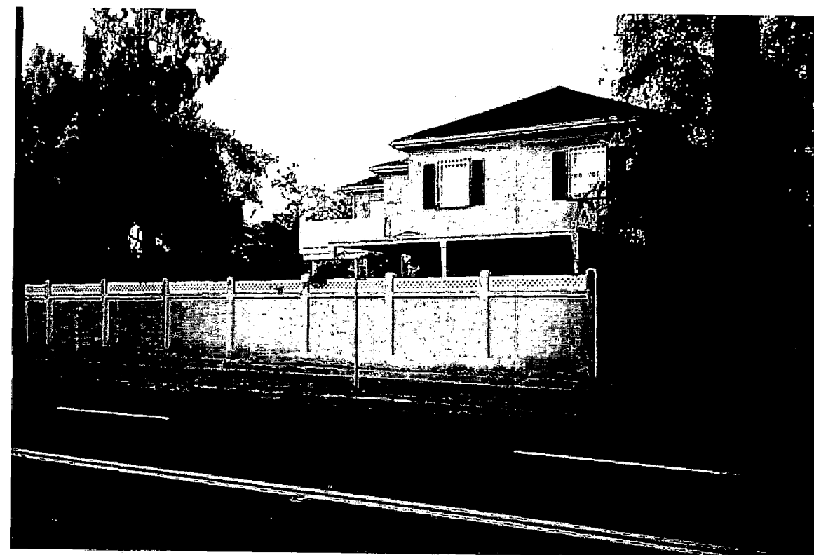
Fence at 44 th and J Streets, Height 93 ½" with No Street Side Setback
