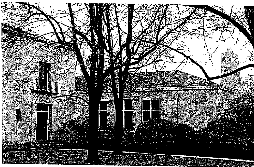
Figure 3 Sierra School South entry and south wing view southeast
