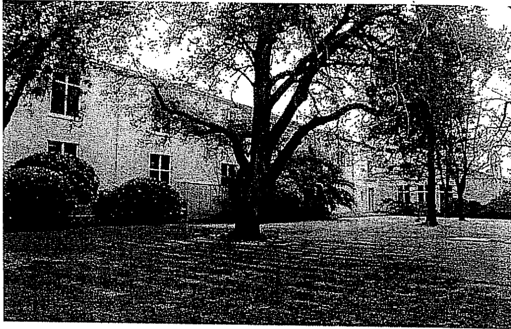
Figure 2 Sierra School Front façade and south wing view southeast
