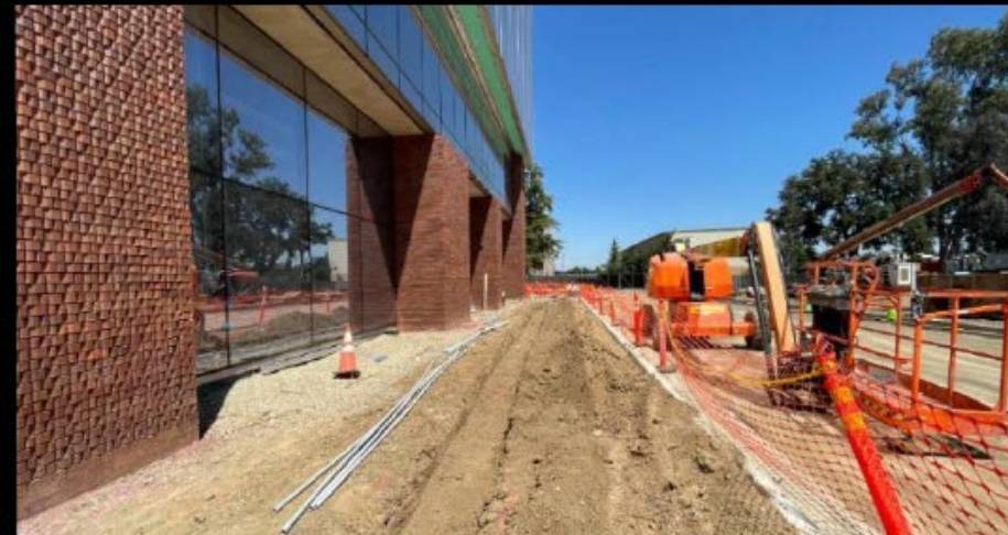
Excavation for Site Lighting
