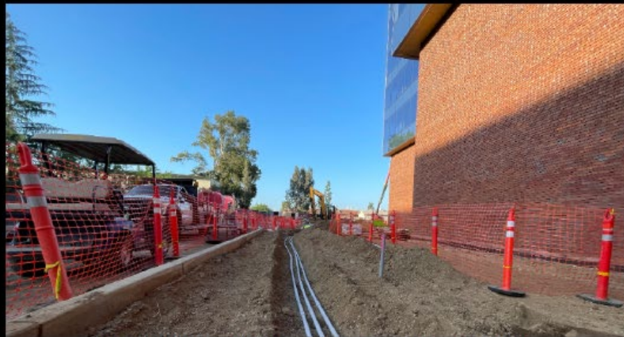
Installed Conduit Home Runs Southeast of LLL
