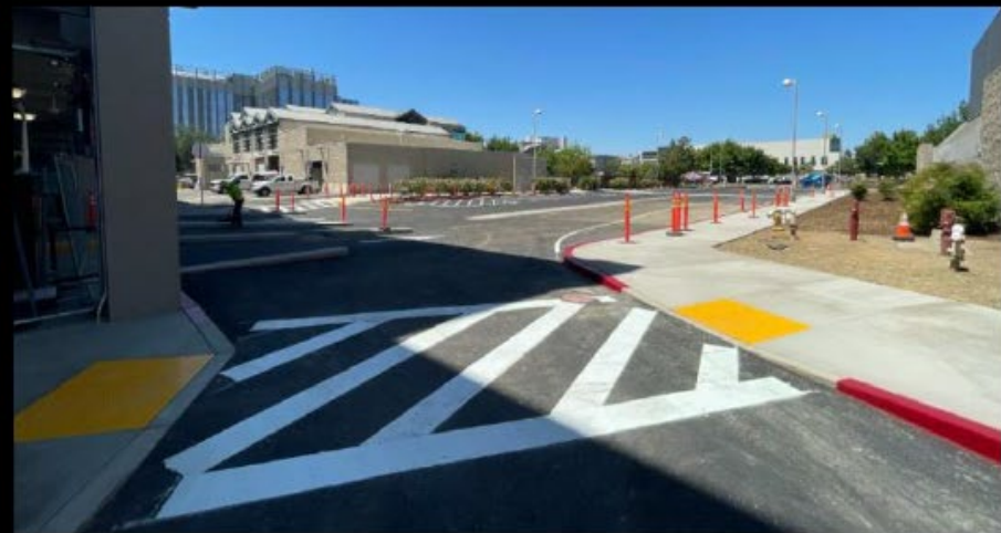
Concrete Ramps Placed by PS6
