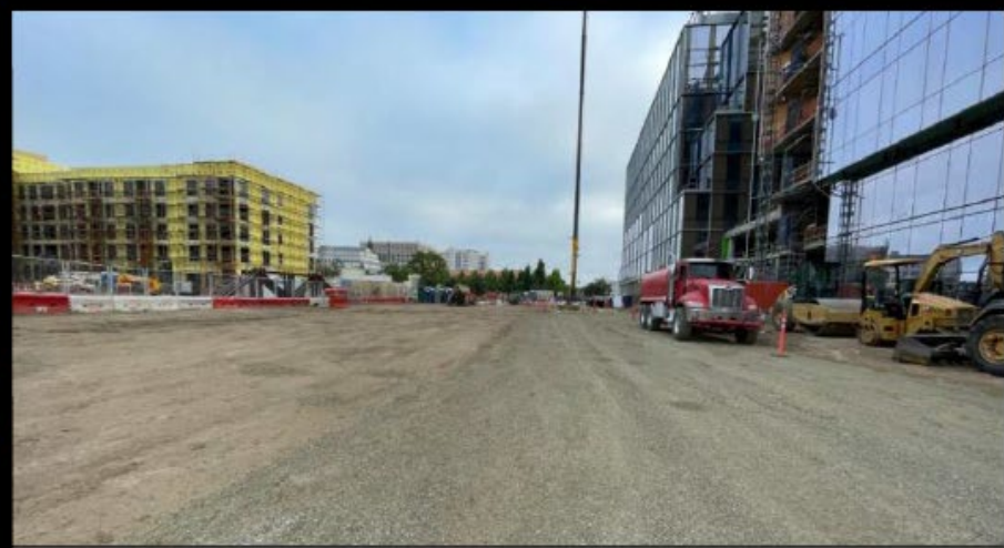
Placed AB in Road Section on Paseo
