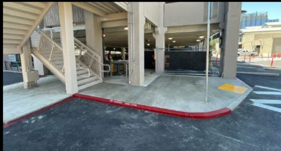
Flat Work Completed by PS6
