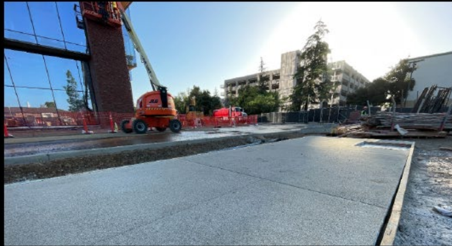
Concrete Sidewalk Mock-Up Review
