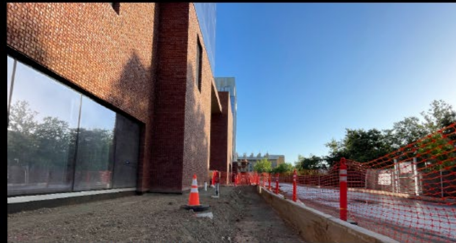
Excavated for Planter Boxes on the Southeast Corner of LLL
