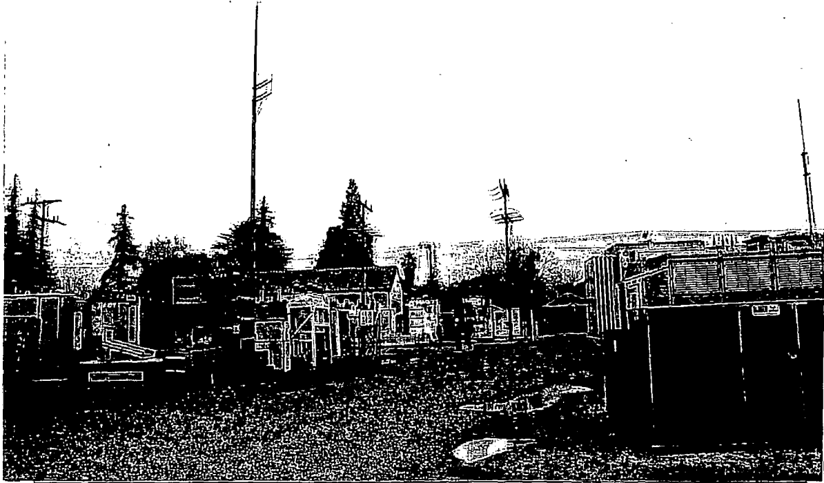
VIEW FROM SOUTH SIDE OF FACILITY
