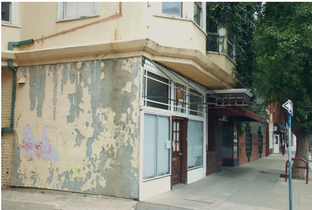
Retail storefront on south side. View to northwest.
