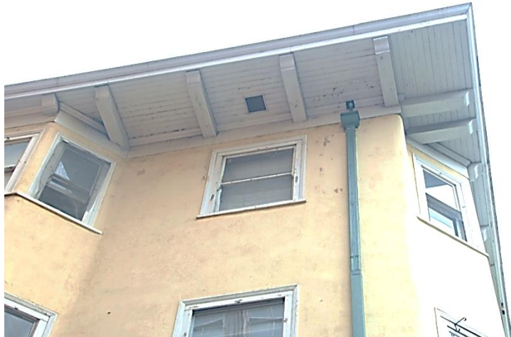
View of mean detail in soffit.
