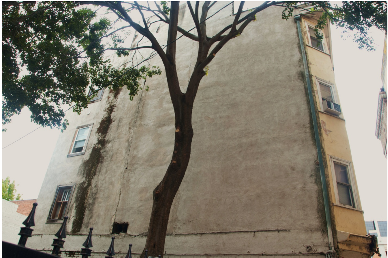
Rear building elevation. View to the east.
