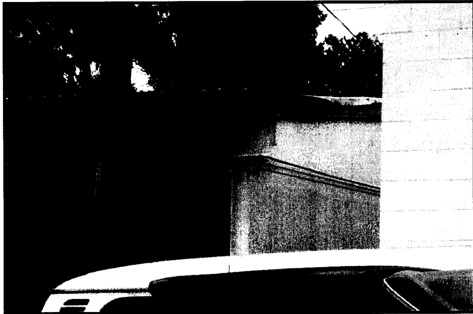
Photo 4: 5900 Elvas Avenue. This building is suffering from deterioration to the roof and eave. The eaves are left exposed subjecting the building to dry rot and undermining its structural integrity.
