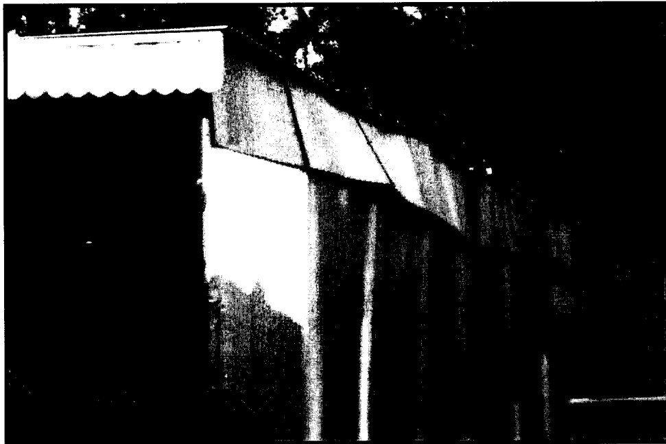
Photo 5: 5900 block of Elvas Avenue. This structures corrugated walls are deteriorating and separating from the building, subjecting the bearing wall/structural support to deterioration.
