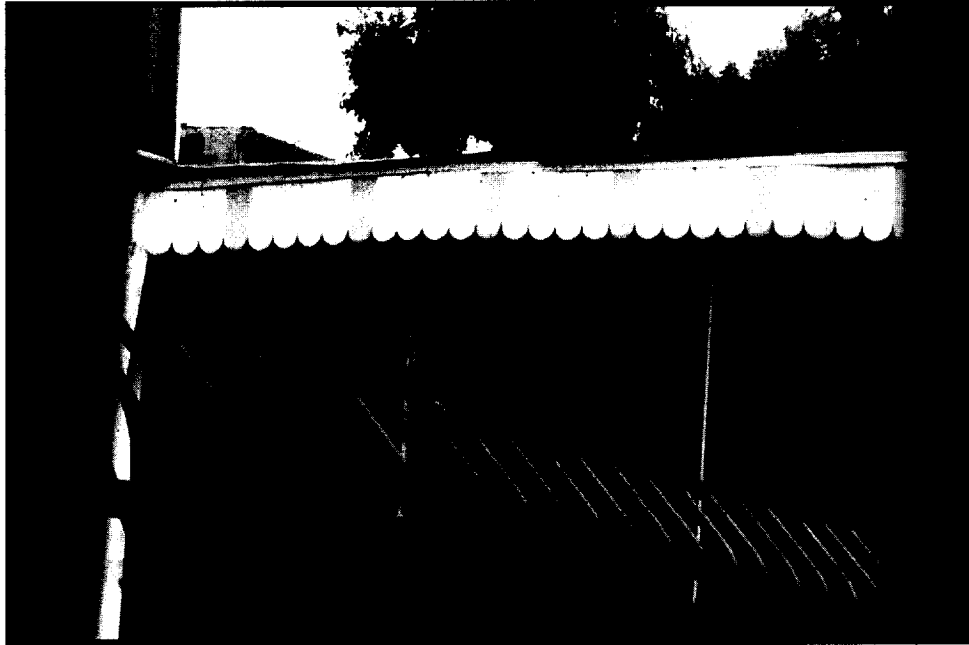
Photo 6: 5900 block of Elvas Avenue. This structures roofing and wall material is deteriorated. The structural support, rafters, and eaves are completely exposed and there are gaps between the wall and roof. Additionally, the roof and portion of wall are constructed with corrugated metal.
