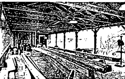
Much of the construction takes place in the 20 x 60 shed constructed next to the ship. The seaward end of the shed contains the yard office.
