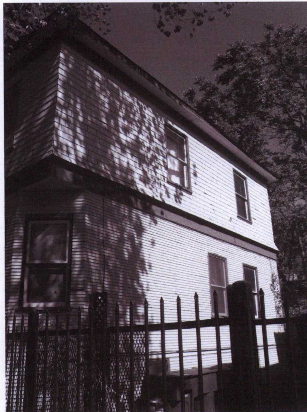
1905 "I" Street, East Elevation including wood shingle and drop siding, framed by wide trim pieces, including under the soffit
