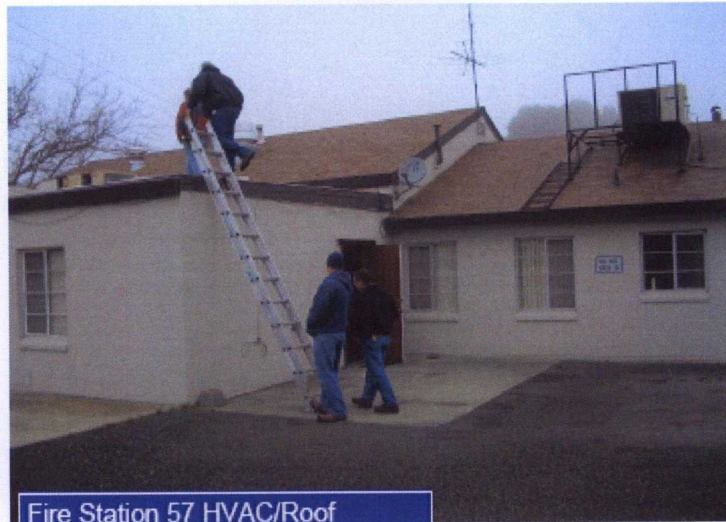
Fire Station 57 HVAC/Roof
