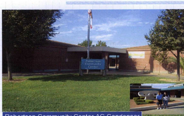
Robertson Community Center AC Condenser
