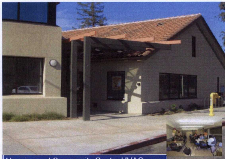
Hagginwood Community Center HVAC
