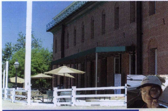
Discovery History Museum Fire Alarm System
