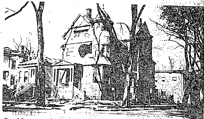
85/24/373 Residence of Col. H. Weinstock.. "1630 H street". Next door, "1623" H. st...Building erected in 1893...In the 1880's, horse-cars "rolled" by this place.
