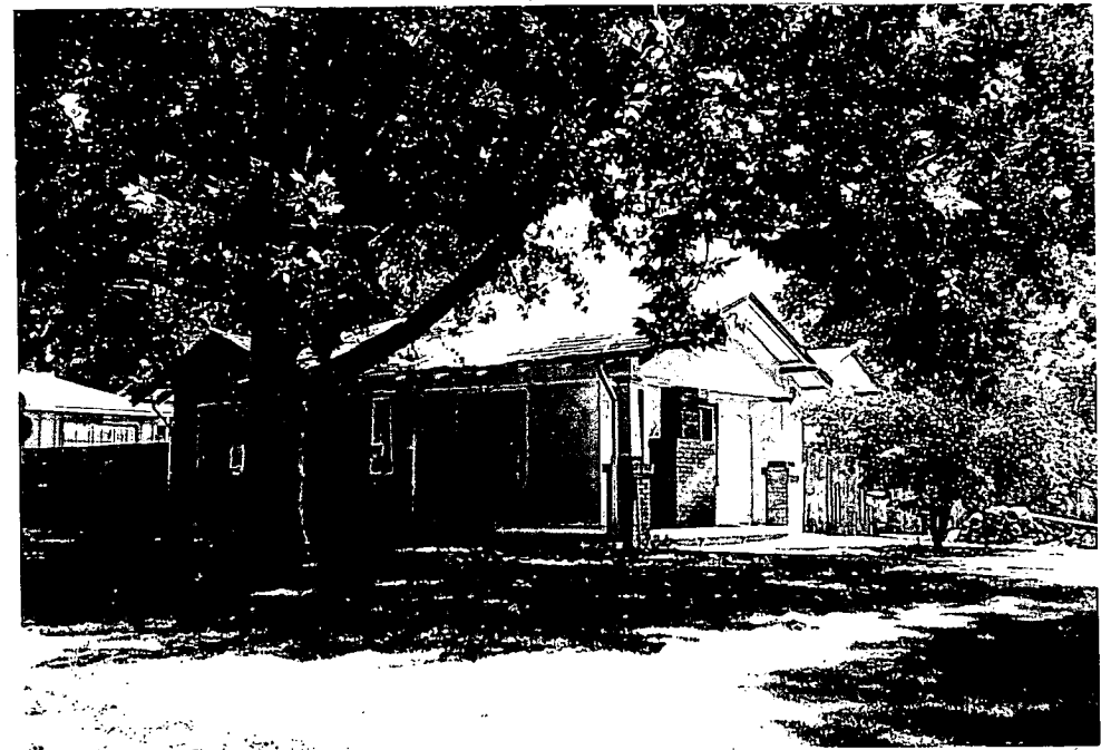
of Existing house 3406 Ivy St
