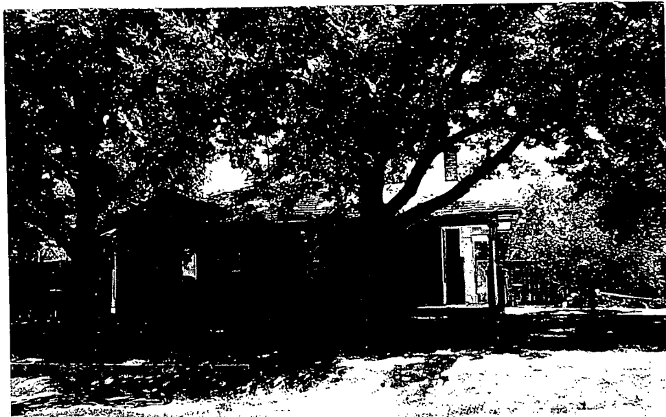
EXISTING HOUSE 3406 IVY STREET
