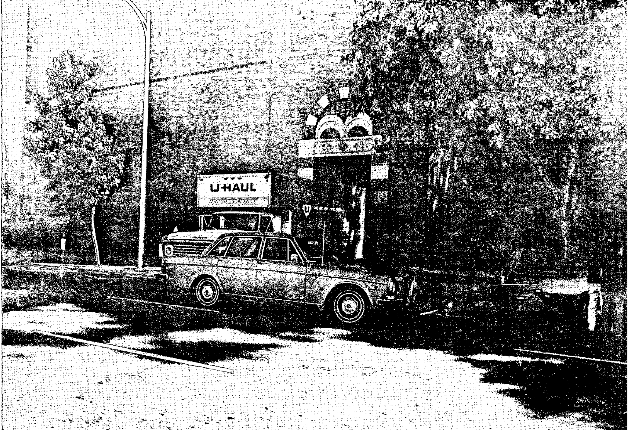
STAGE DELIVERY DOORS AT J STREET. PROPOSED WORK WOULD PROVIDE AN ON-SITE TRUCK DOCK AND EFFECTIVELY ELIMINATE VEHICULAR AND PEDESTRIAN HAZARDS.
