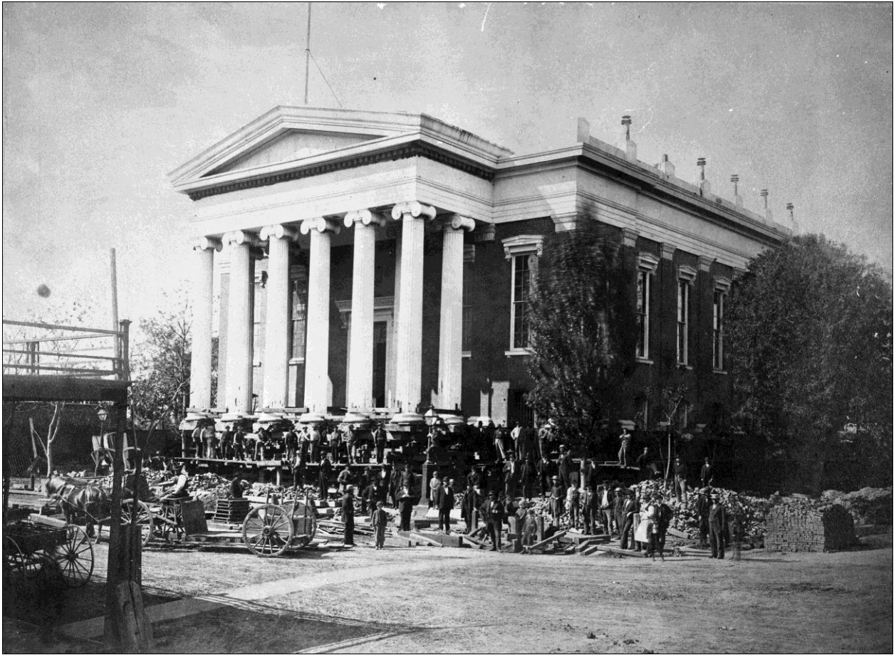
Figure 16. To avoid floodwaters, many buildings in Sacramento were raised in the 1860s and '70s. Pictured is the Sacramento County Courthouse being raised with jacks.
