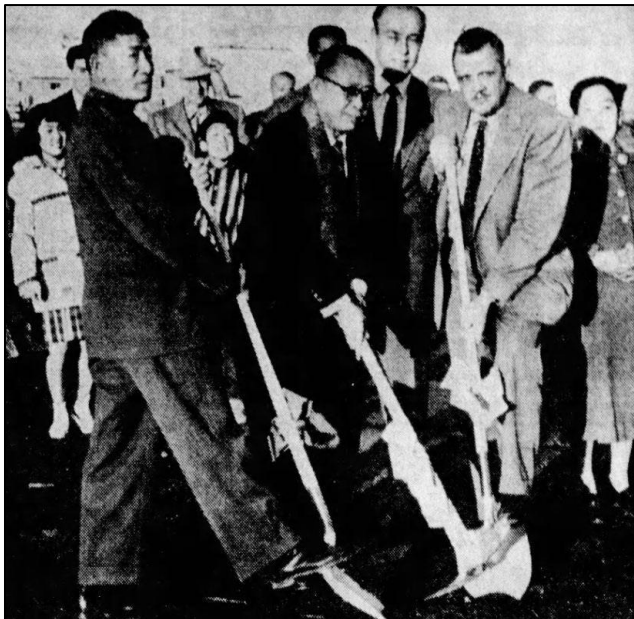
Owner Gonzo Sakai, Rev. Senshow Sakai and the Warren brothers breaking ground, 1960 (Sacramento Union).
