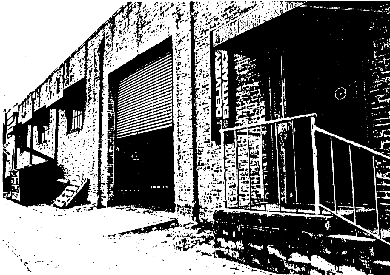
A) Unreinforced masonry structure on Barstow Street between Del Paso Boulevard and El Monte Avenue.
