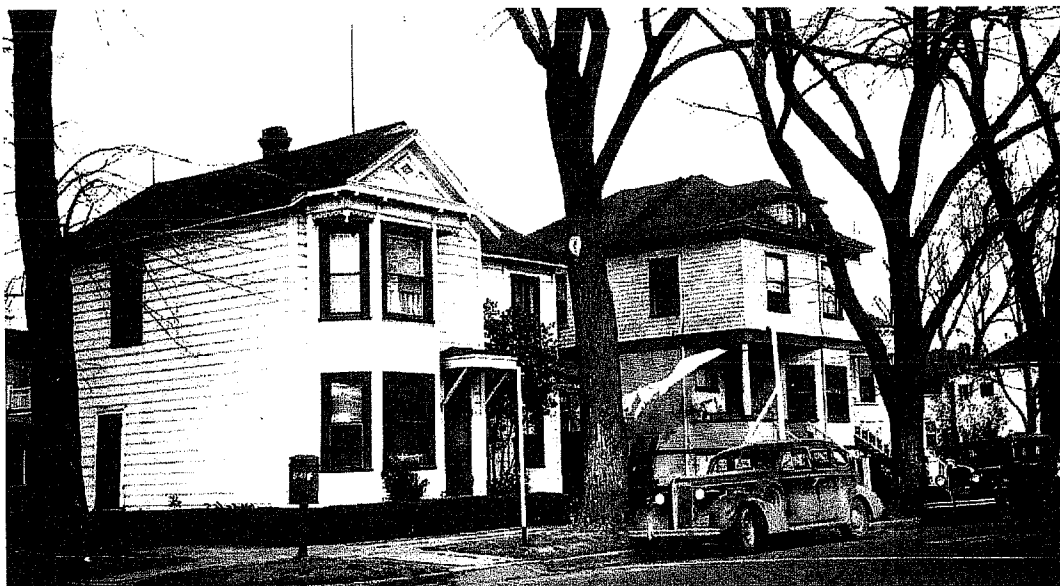
This 1949 photo by Eugene Hepting shows 1901 and 1905 I Street. The owner plans to return the porch to its appearance in this picture. That plan includes the turned post, enclosed balustrade, front steps and the open balustrade on the steps.
