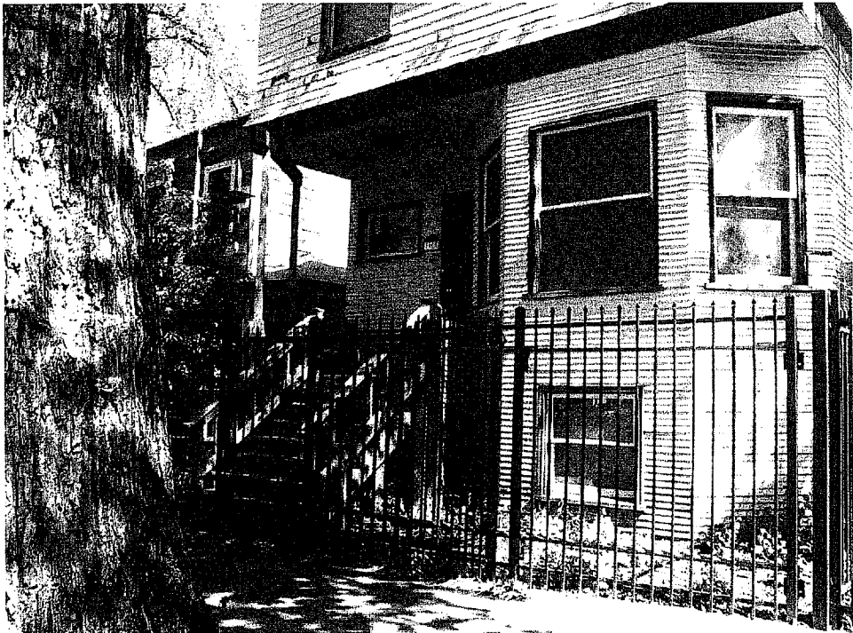
1905 "I" Street, recessed front porch and angled front bay
