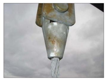
PHOTOGRAPH 6 – Wire suspender rope at top socket connection in good condition.
