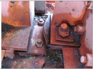
PHOTOGRAPH 5 – Fixed bearing detail and bulging elastomeric bearing pad.
