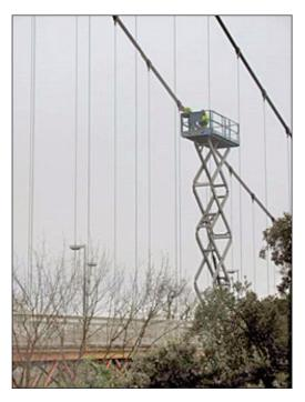
PHOTOGRAPH 2. Access to towers and upper portions of the suspension cables and vertical suspender ropes gained using an 86-foot aerial boom lift.
