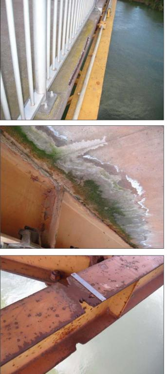
PHOTOGRAPH 1 – Spalling of the deck panel edge beyond the handrail. Note the exposed reinforcing bar.
