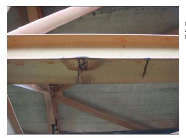
PHOTOGRAPH 4 – Impact damage to the north approach truss lower chord bottom flange between L4' and L5'.
