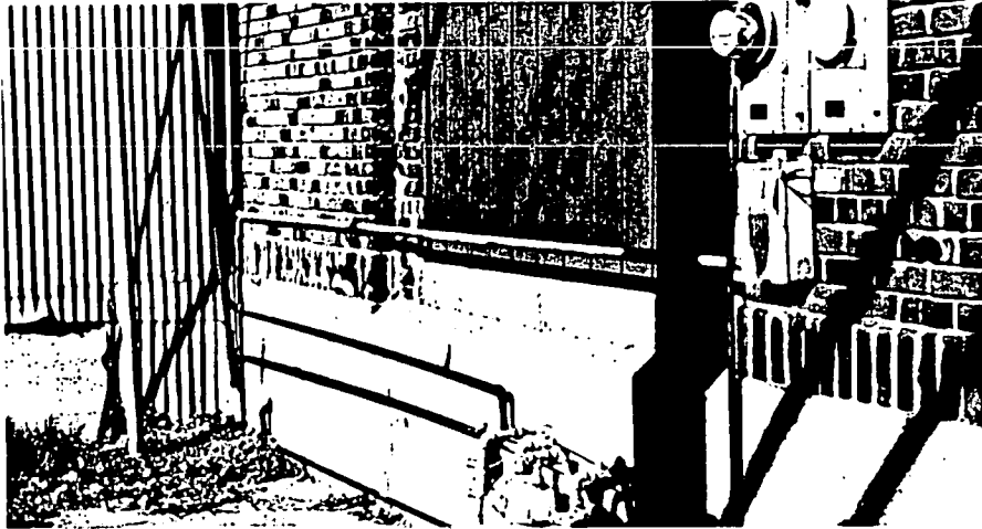
Exposed, deteriorating utility boxes/piping.
