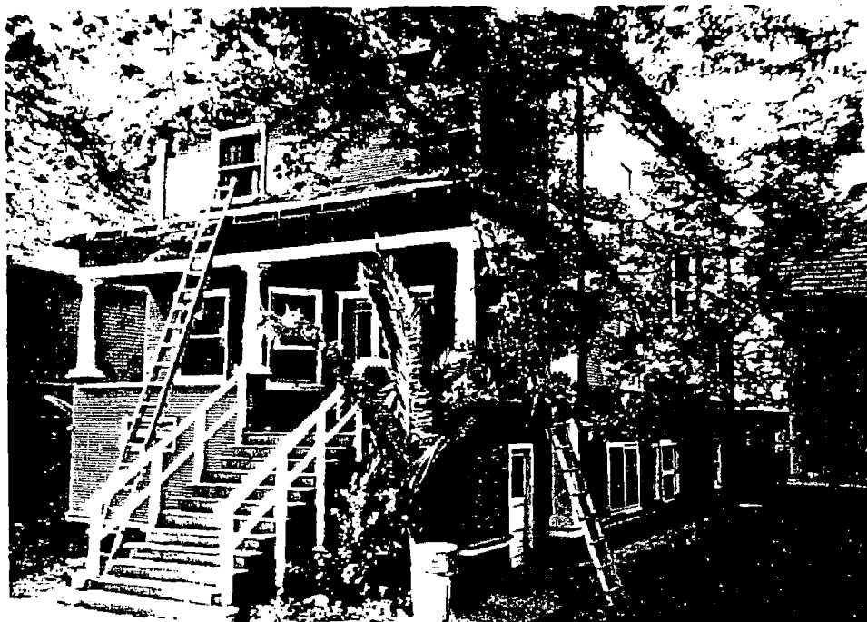
Please note: This photo was taken during repairs.
