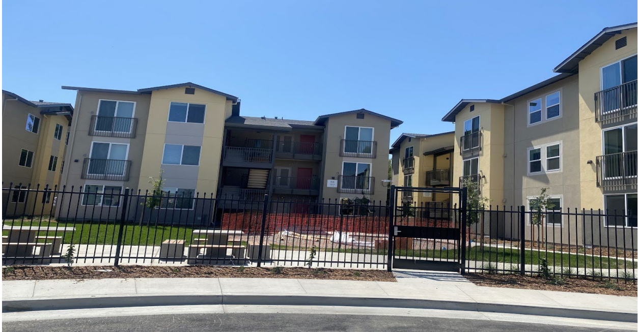
Pictures of Coral Gables (New Construction Site on Vacant Lot)
