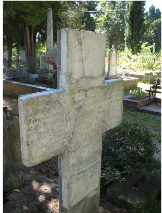
Figure 10- A fractured gravestone has been repaired using a stone backing.
