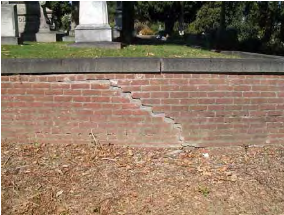
Figure 13- (Left). A large crack in a brick retaining wall. (Right) The brick wall has open joints, particularly near the ground surface.
