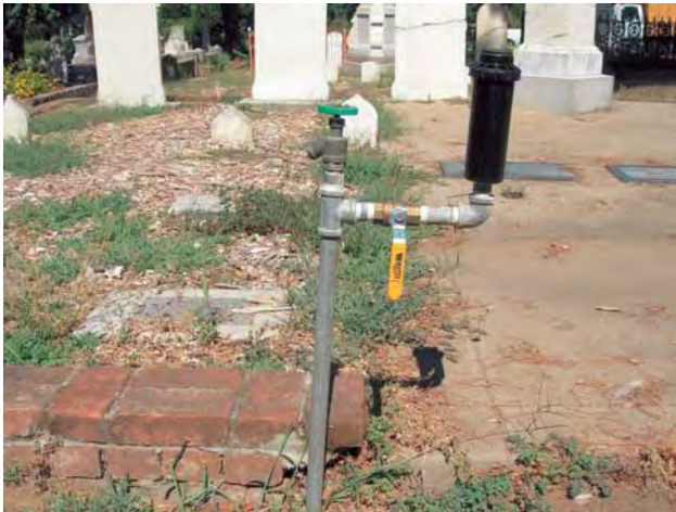
Pop-up head on fixed riser with manual valve.
