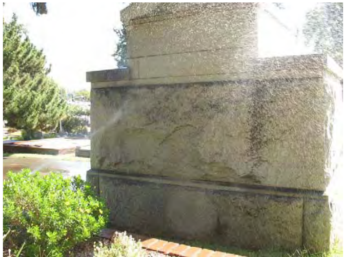
Figure 20-Many of the sprinkler heads are set to directly impact the monuments at close range, causing excess exposure to moisture.
