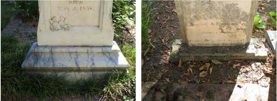
Figure 7- (Left) A gravestones set on a new stone base. (Right) A gravestone set on a concrete base.
