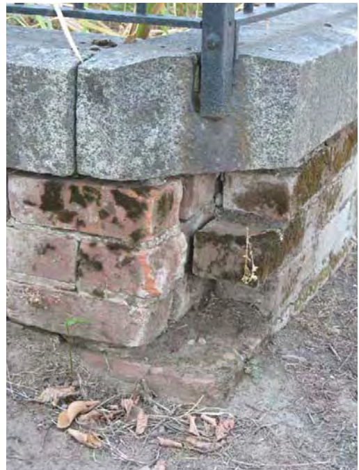
Figure 15- (Top) Much of the ironwork is corroding. (Bottom) The iron fencing expanded as it corroded, cracking the stone.
