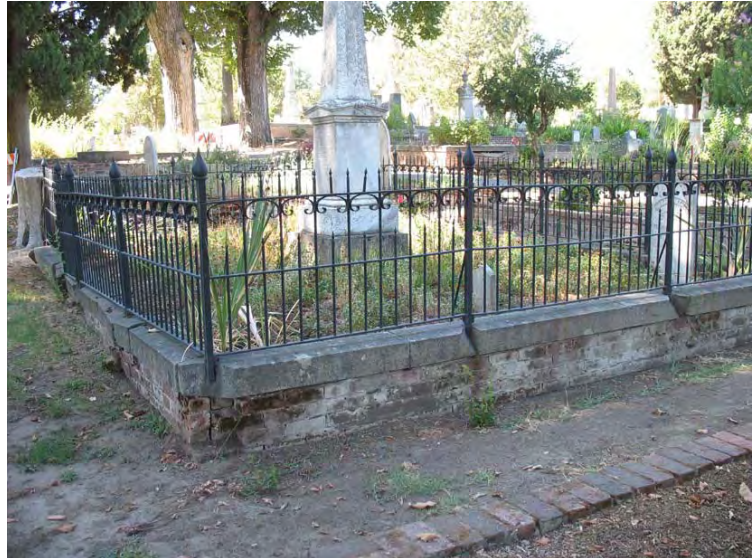
Figure 16- (Top) Originally the fence was set on a masonry base. (Bottom) As the masonry cracked, the base was likely removed and the fence set onto the ground.
