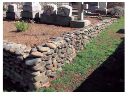
Mortared river rock burial plot wall
