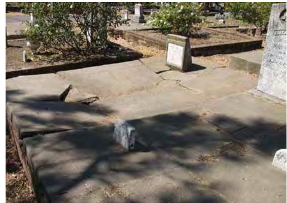
Figure 14- The concrete slab has cracked and failed.
