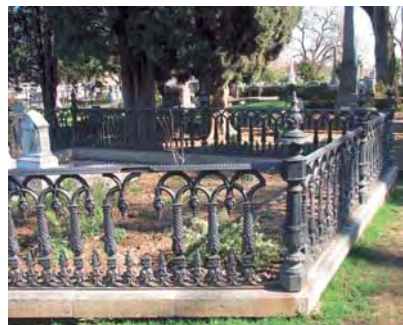
Stone plot enclosure with cast iron fence
