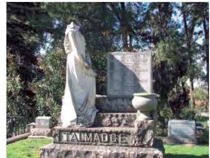
Damaged and Delaminating Monuments
