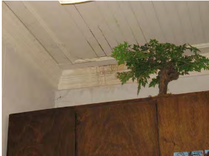
Figure 3- Water staining on the ceiling of the Mortuary Chapel gives evidence of water intrusion.
