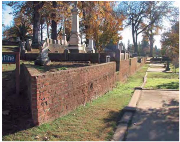
Brick retaining wall for terrace
