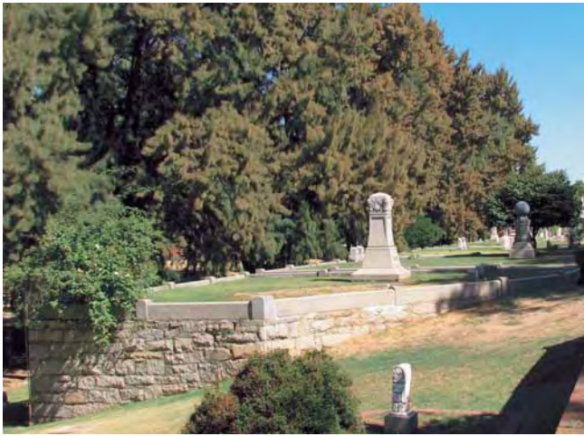
Stone retaining wall for terrace
