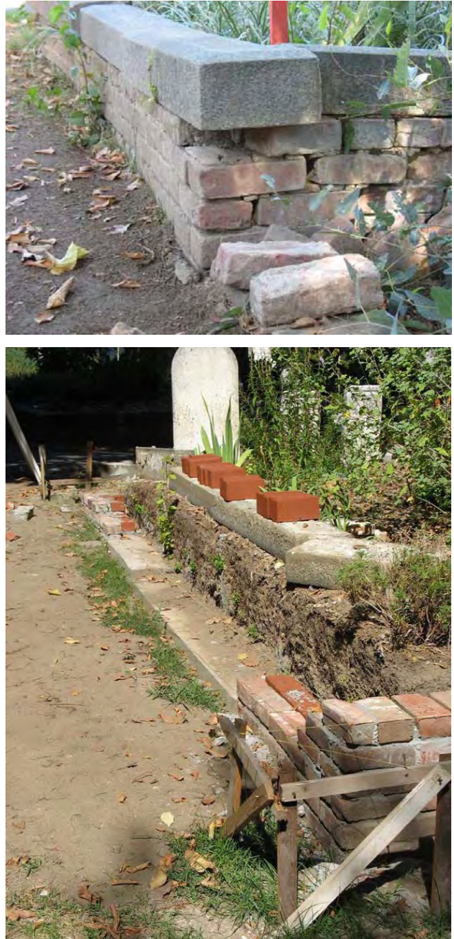
Figure 12- (Top) The brick is dislocated and joints are in poor condition. (Bottom) A brick enclosure currently being rebuilt with a new concrete footing.
