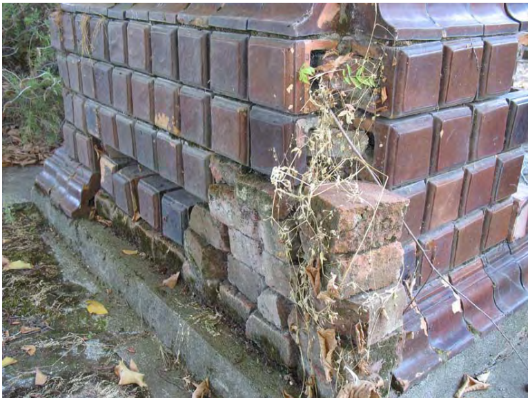
Figure 11- The Georgia Fisher monument with missing masonry units.
