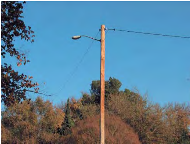
Not appropriate - overhead wires and cobra-head lights
