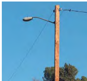
"Cobra Head" Light Fixture
