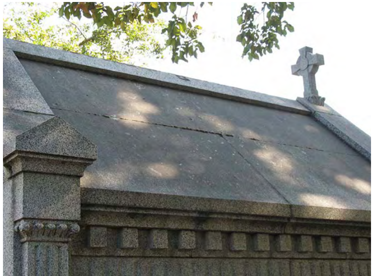
Figure 4- Well maintained masonry joints are critical to keeping the masoleum watertight.
