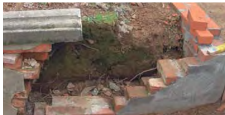
Brick Deterioration
