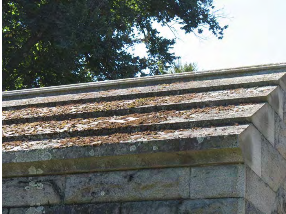
Figure 18- Excess biological growth is present on the roof of the masoleum.
