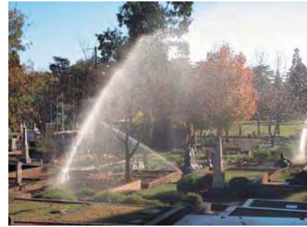
Existing High-Impact Spray Rotors
