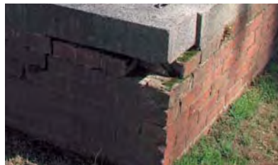
Brick Deterioration
