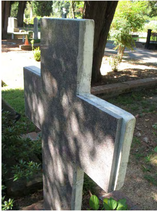
Figure 10- A fractured gravestone has been repaired using a stone backing.
