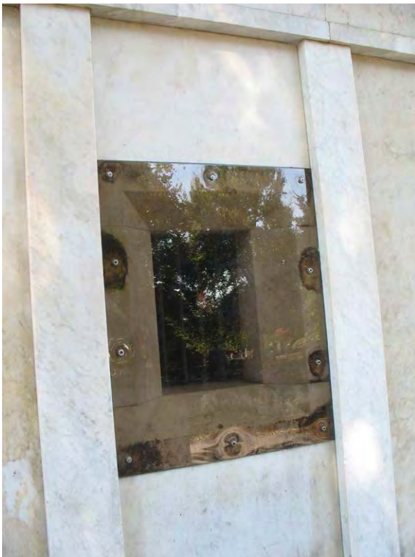
Figure 17- The protective plastic is unvented and biological growth is evident on the interior surface.
