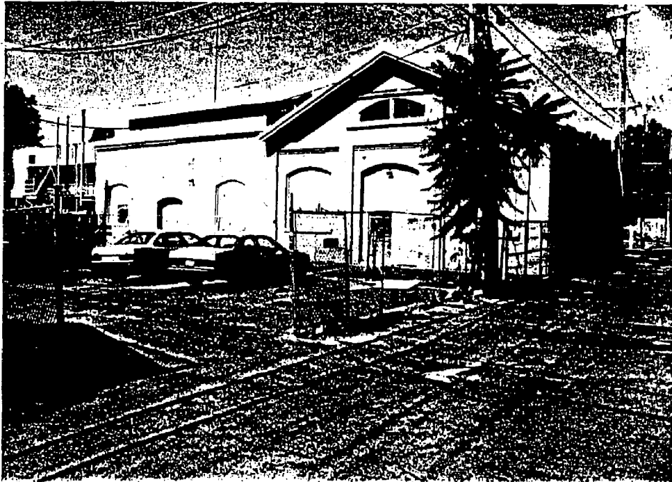
Looking west across the alley at the back and north sides of the building.
